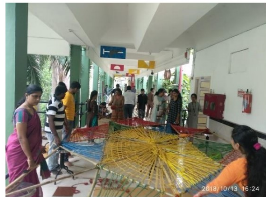
Completion of Bamboo Roof on 13-10-2018 @E210 - School of Architecture
